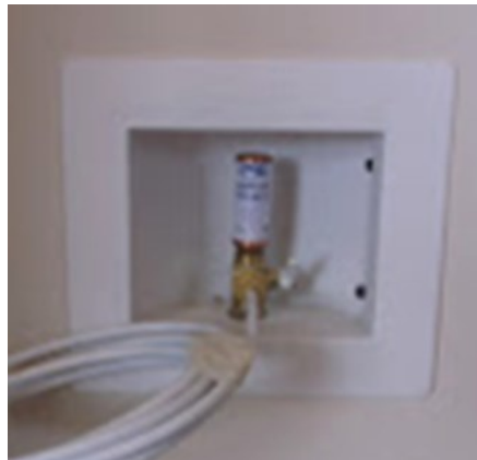
PLUMBING PREP FOR ICE MAKER WITH WATER HAMMER ARRESTORS
