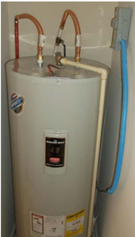
50 GALLON ROUND TALL ENERGY SAVER ELECTRIC WATER HEATER
