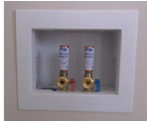
PREP FOR WASHING MACHINE WITH WATER HAMMER ARRESTORS
